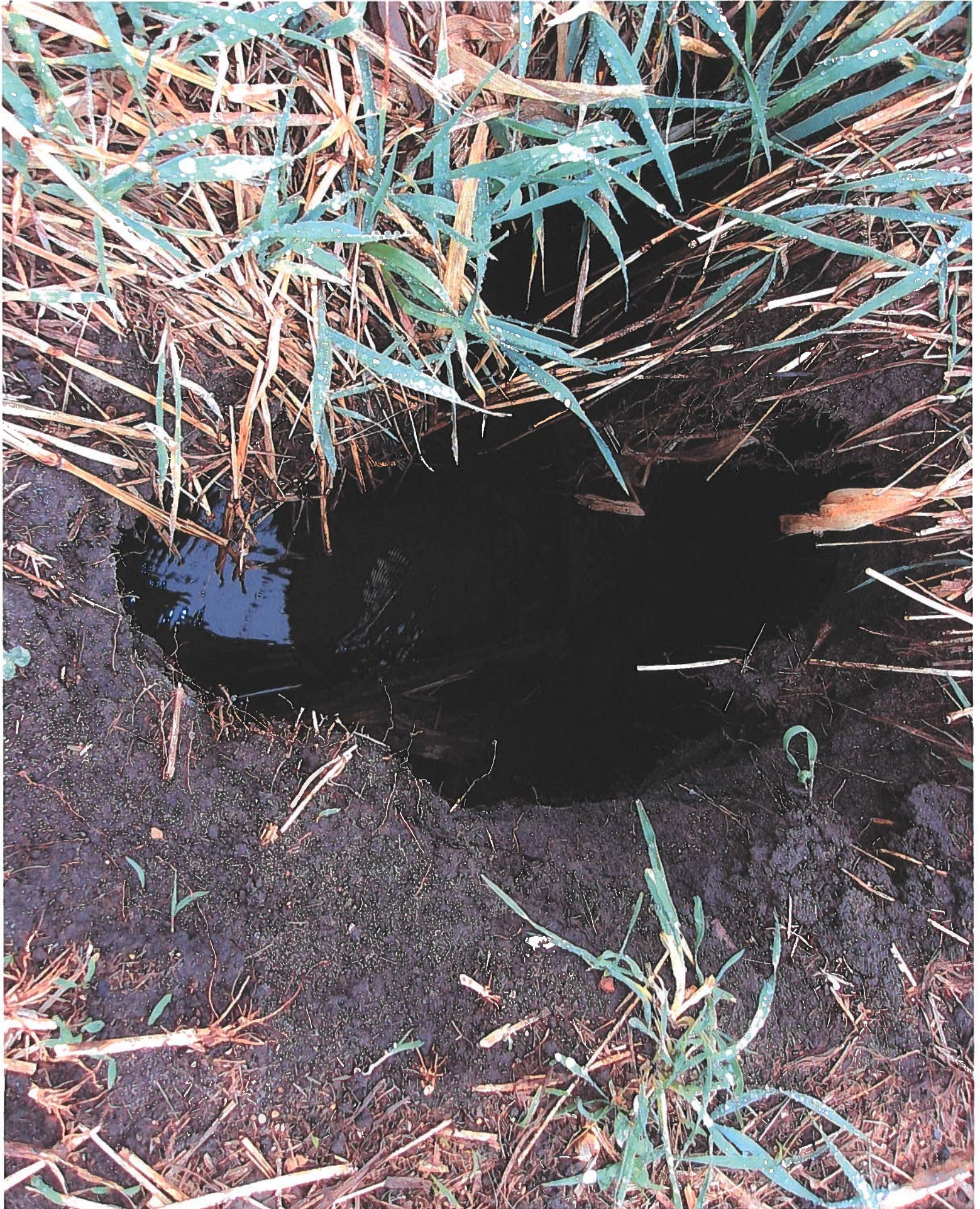
Collapsed Clay Tine
